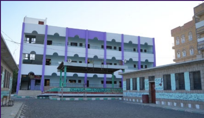
Ali Bin Abi Taleb School after rehabilitation.
